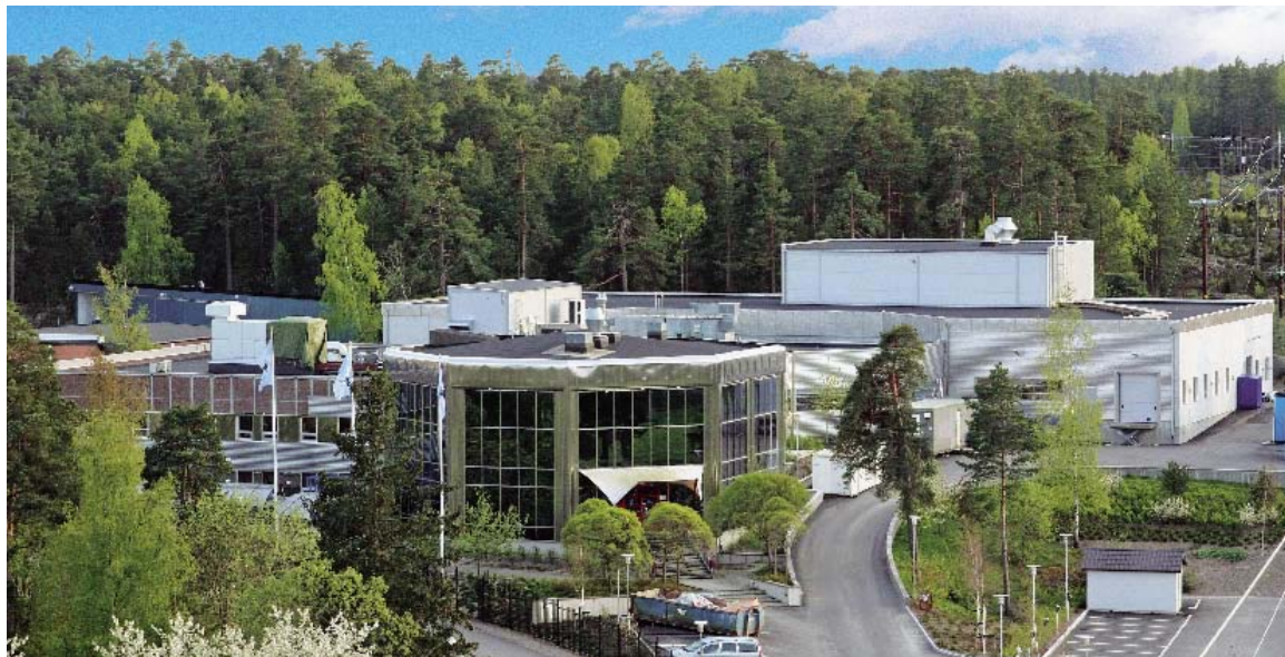
The white building in the background is the latest addition. The box on the roof contains the air and water cleaning equipment. The water is pure H 2 O. It is ultraclean and is used during manufacture for washing and humidifying the air.
